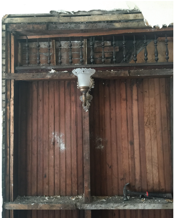
Woodwork hidden inside of a plastered wall. Sconce addition by Laine.
